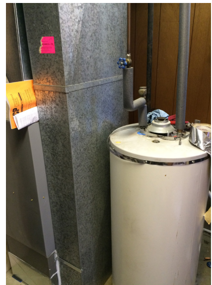
Figure 2: ‘Orphaned’ hot water tank
